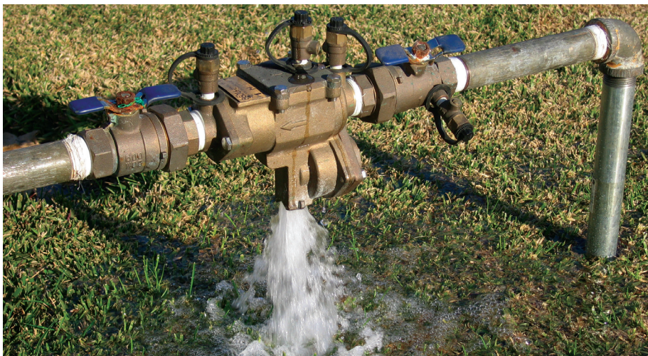
Reduced Pressure Principle Assembly with leaky relief valve
